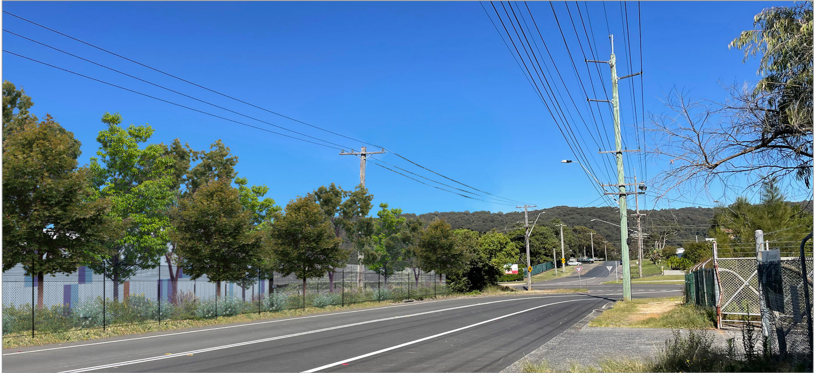
MONTAGE VIEW WEST ALONG FAUNCE STREET WEST -Towards the intersection of Young Street
